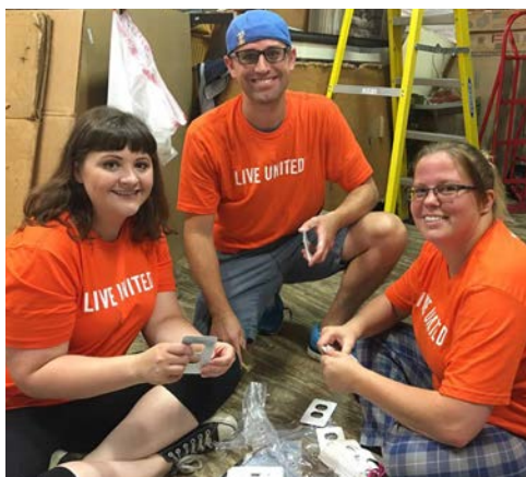
No detail is too small for Caitlin Kelly (left), Nick Piper (center) and Holly Bresson (right), who unpack new wall plates complement the new coat of paint.
